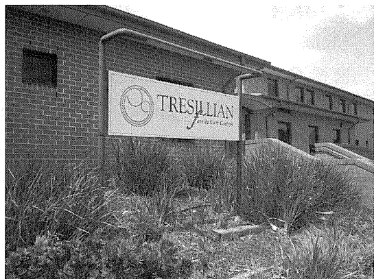
写真2 Tresillian Family Care Centre, Canterbury
