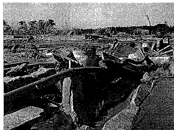
Photo 4 Damage to pipe by scouring of tsunami (Miyagi Pref.).
