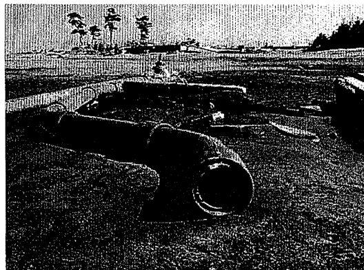
Photograph 4 Damage to pipe by scouring of tsunami (Miyagi Pref.).
