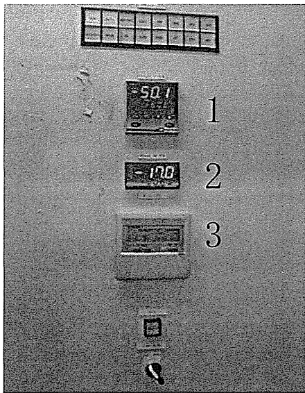
Fig. 4. Operation mode display. 1: P3 room pressure, 2: Ante-room pressure, 3: Temperature display
