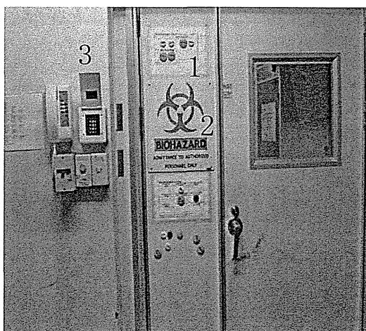
Fig. 15. Multiple signage. 1: Activated pathogens symbol, 2: Biohazard sign, 3: Lock pad (a security feature)
