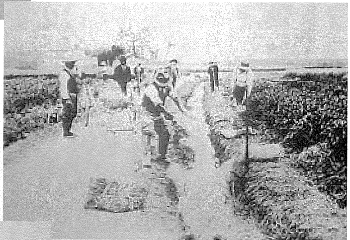
Figure 39. Application to the canals of quicklime.
