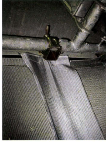
Photo 5. A small piece of sheet fixed onto plastic sheets to add strength
