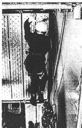
(a) Prefabricated scaffolds.
