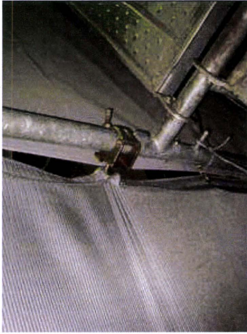
Photo 2. The plastic sheets bound to the pipe of the scaffolds by exclusive coupler
