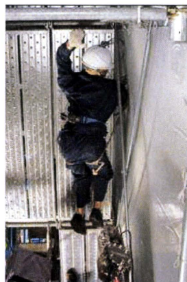
(b) Prefabricated scaffolds
