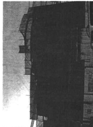
Photo 1 Scaffolds covered with plastic sheet
