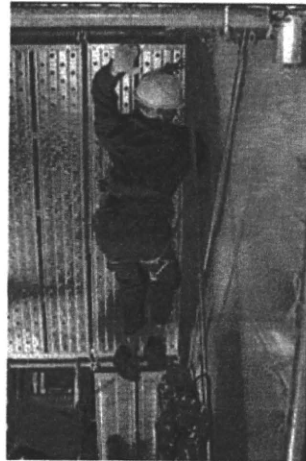
Photo 2 Typical prefabricated scaffolds used in Japan
