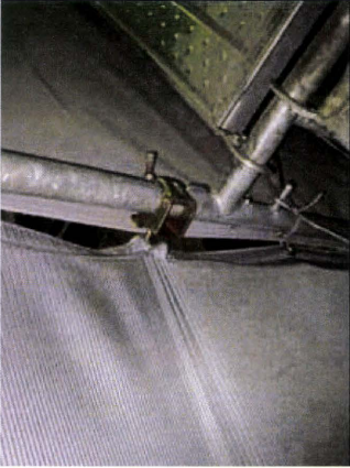
Photo 4. The plastic sheets bound to the pipe of the scaffolds with a special coupler.
