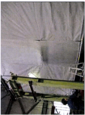
Photo 4. The plastic sheets bound to the pipe of the scaffolds with a special coupler.
