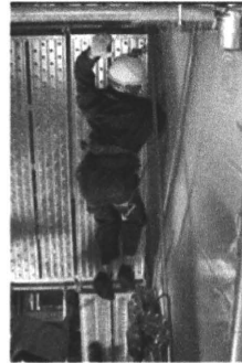
Photo 2. Typical prefabricated scaffolds
