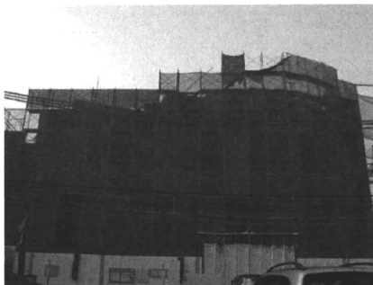
Photo 1. Scaffolds covered with sheeting
