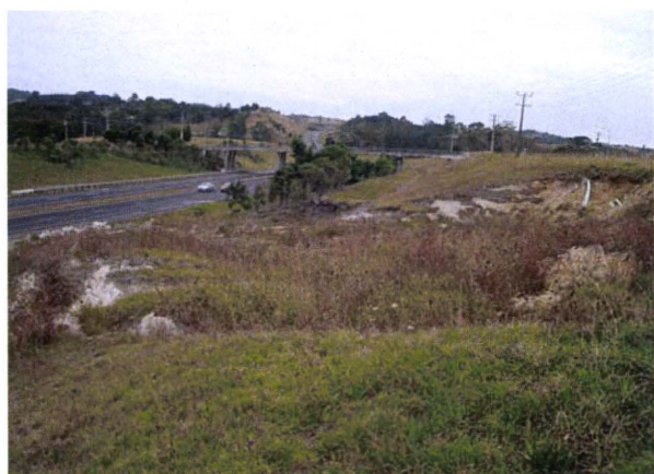
Figure 1. The monitored site. The landslide occurred in the winter of 2008. State Highway 1 can be seen at the toe of the slope.
