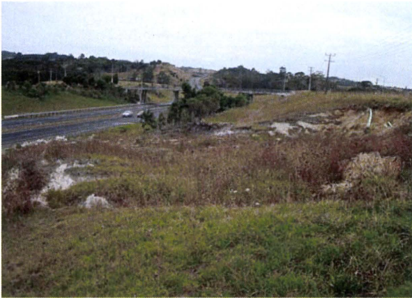
Figure 1. The monitored site. The landslide occurred in the winter of 2008. State Highway 1 can be seen at the toe of the slope.
