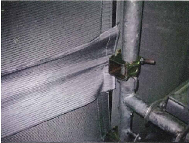
Photo 7. A small piece of sheet fixed onto plastic sheets to add strength.
