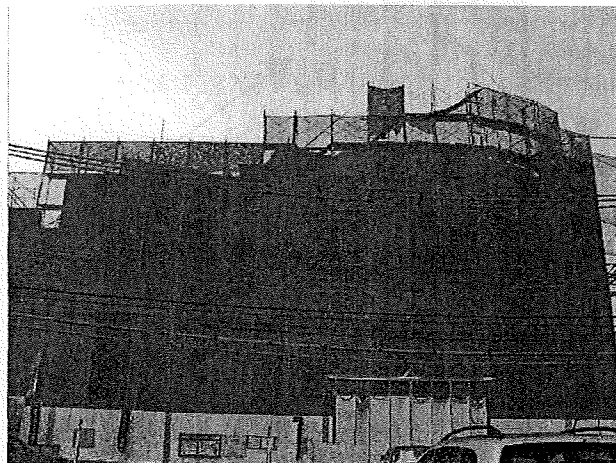
Photo 1 Scaffolds covered with plastic sheet
