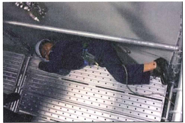
(a) Pipe scaffolds.
