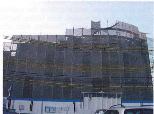
Photo 1 Scaffolds covered with mesh sheet.
