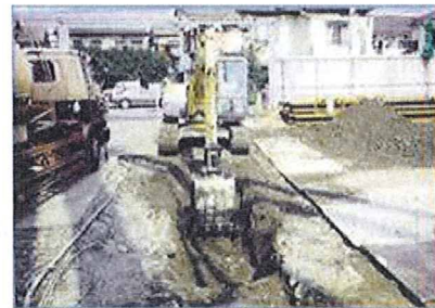
FIG.3. Preliminary trench excavation.
