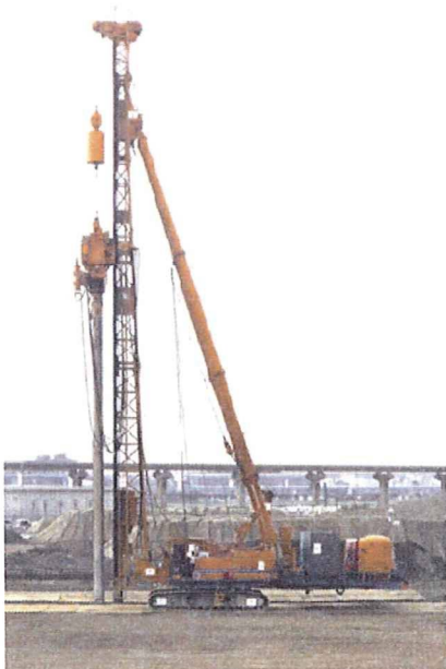
Photo 1. Automotive pile driver
