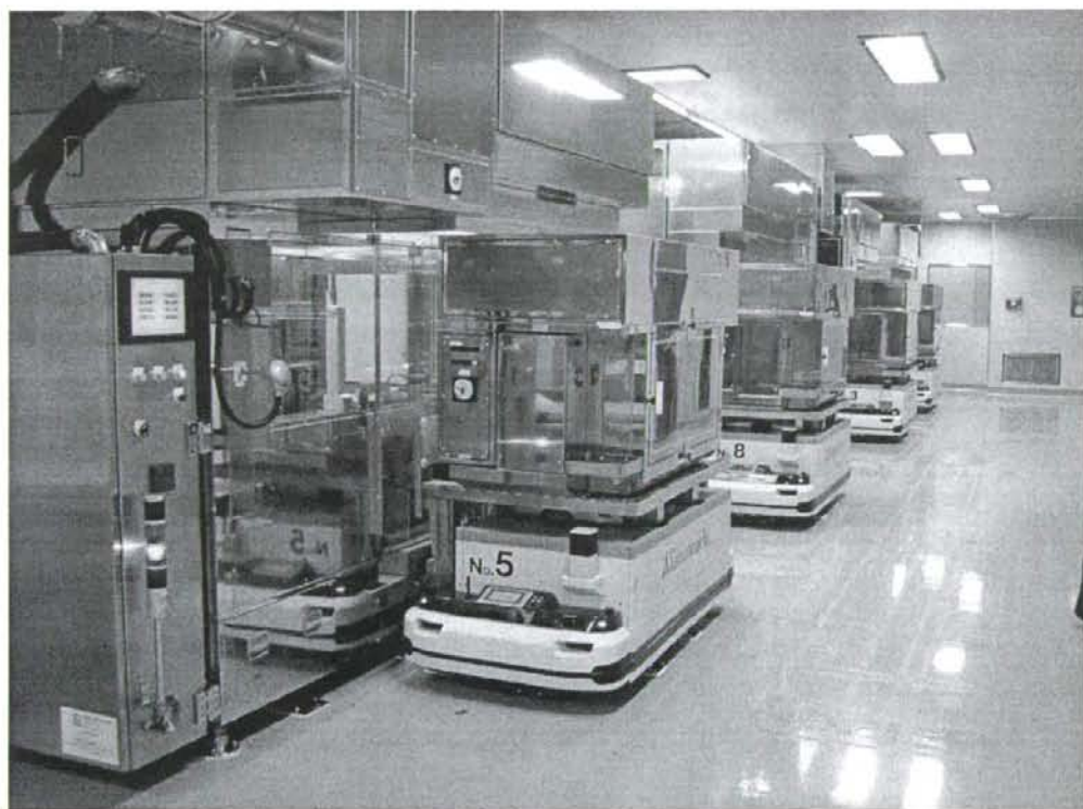
Fig. 9 AGV station for lyophilizers in aseptic area
