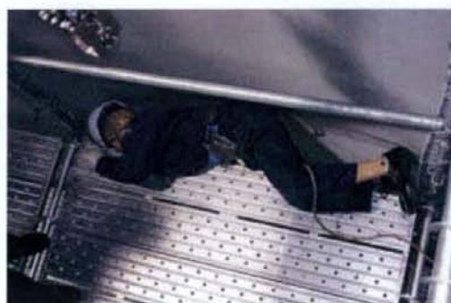
(a) Pipe scaffolds
