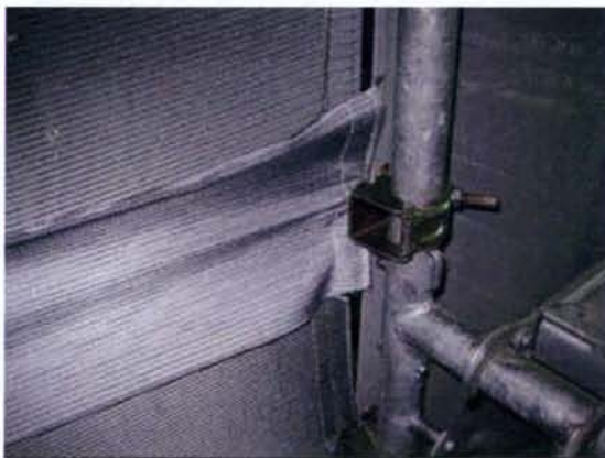
Photo 5. A small piece of sheet fixed onto plastic sheets to add strength
