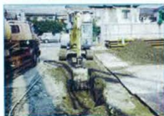
FIG.3. Preliminary trench excavation.
