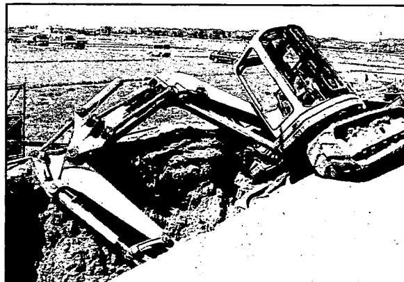
Photograph 1. Ground collapse during trench excavation
