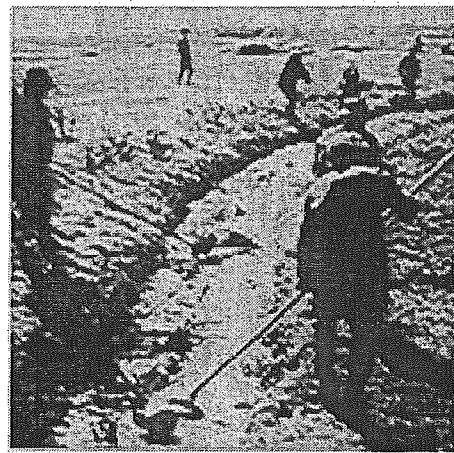
The spread on the side wall of the canal, they used a long arm scraper.
