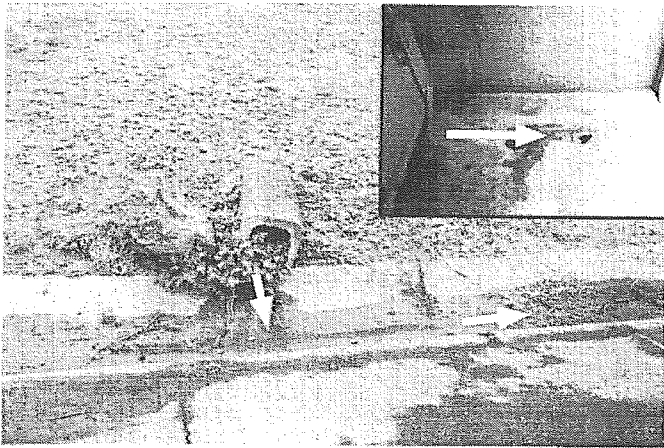
FIGURE 1. Opening site of a waste pipe from a raccoon cote to a shallow drain in the macaque/bear area. The insert photograph at the upper right corner shows the opening of the waste pipe in the raccoon cote. Directions of water flow are indicated by arrows.
