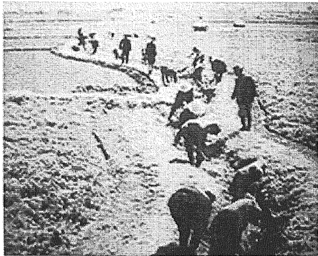
Scraping the edge of the irrigation canals to drop the snails into the water.
