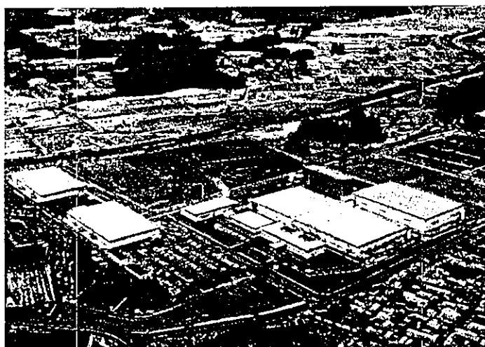
Fig. 16. External appearance of pharmaceutical factory in NIPRO New facilities for the production of artificial oxygen carriers will be constructed in this factory.
