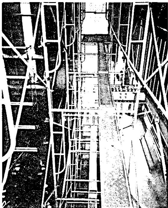
Photo 5 Handrail (cross type). 交差筋交
