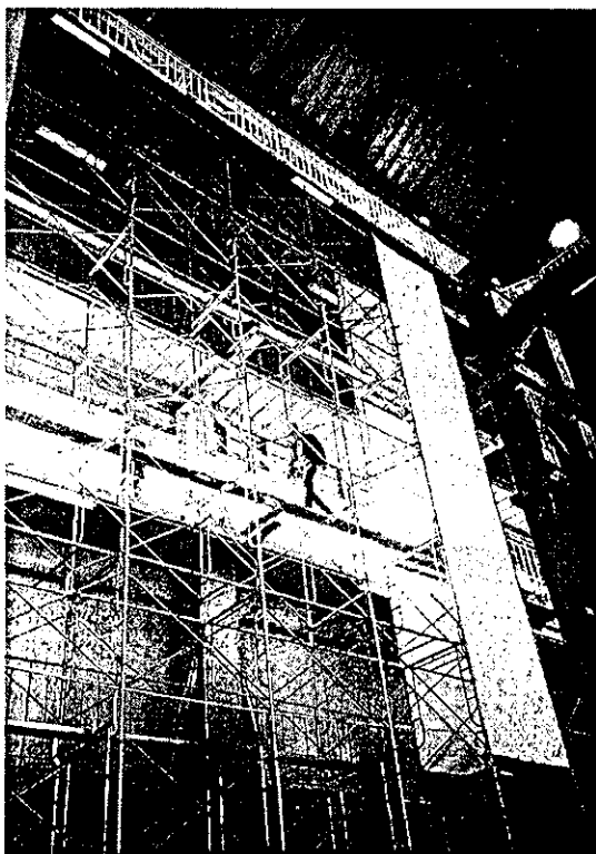
Figure 2. View of the experiment: The test being carried out is at level 4 with a 240 mm-wide footing board.
