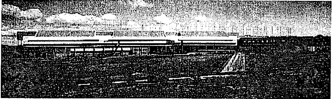
The many "chimneys" along the roof line show how every air handling unit has a separate exhaust, while the air intakes are below the eaves.
